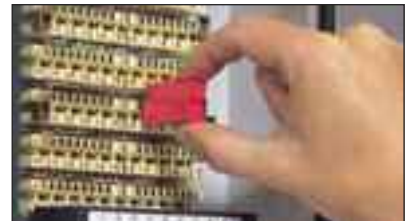
Having pushed the ESP KE10 earth bar on to the disconnection modules' earth points, firmly push an ESP KS06 (or ESP KS15, ESP KS30 or ESP KS50) into each line/pair requiring protection
