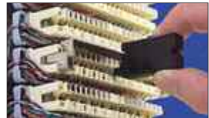
Having pushed the ESP KE10 earth bar on to the disconnection modules' earth points, firmly push an ESP KT1 (or ESP KT2) into each linepair requiring protection
